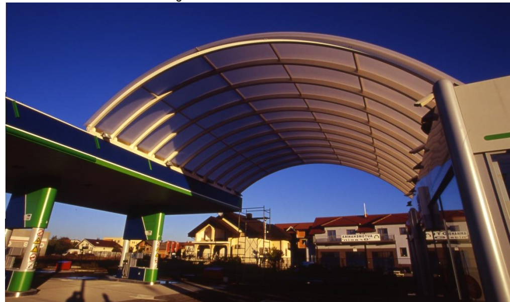
Overhead protection OMV
